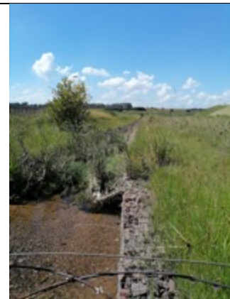
Photo 12: Example of gabions
