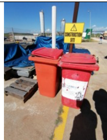
Photo 15: Unlabelled and/ or damaged labelling, Mixing of waste
