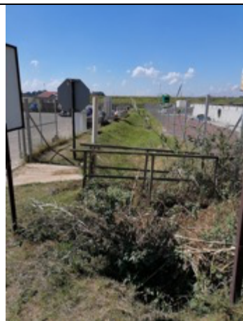
Photo 13: Example of V-trench
