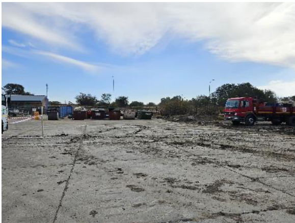
Photo 3: Section outside workshop area with poor waste management, undesignated parking, tyre storage area
