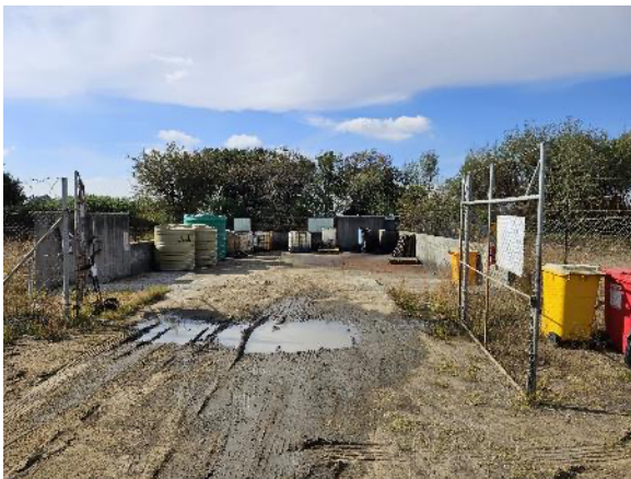
Photo 15: Alien Invasive Species near offices, poor drainage by used oil storage area.
