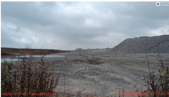
Photo 21: Ponding near hard stockpiles
