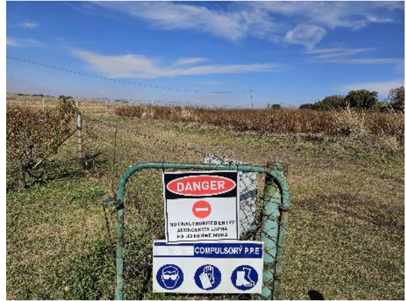
Photo 8: Restriction and safety signage Sewer Plant Office
