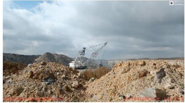
Photo 20: Backfilling by Dragline
