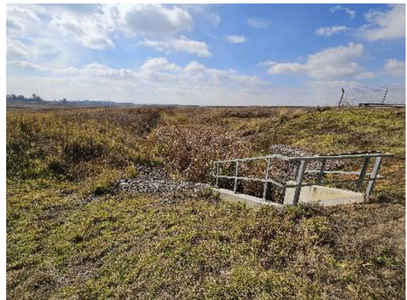
Photo 10: Diversion Water Dam culvert spillway outlet structure, all in good condition, good vegetation growth
