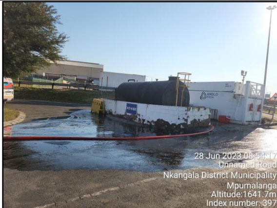
Photo 1: Dust aside tank in a bunded.
