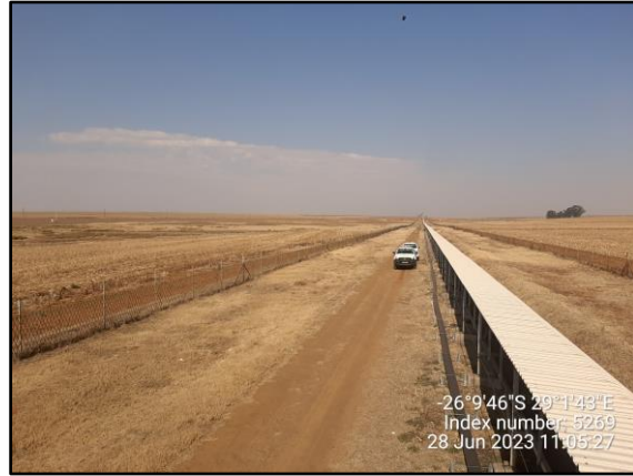
Photo 8: Conveyor belt covered with doghouse sheet.
