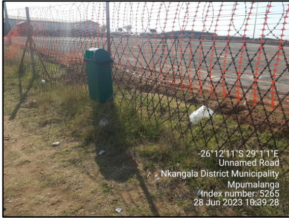
Photo 7: Littering observed at mine.
