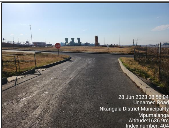
Photo 5: Stop sign erected along the road.
