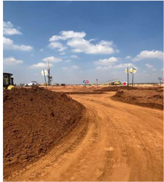
Figure 8: Internal Access Road
