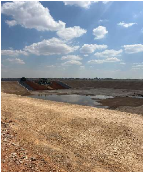
Figure 15: PCD under construction
