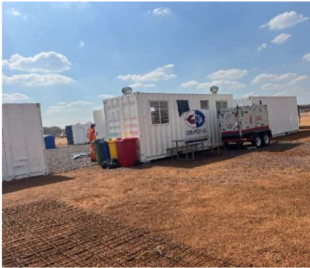
Figure 23: Wheelie bins at contractors laydown area
