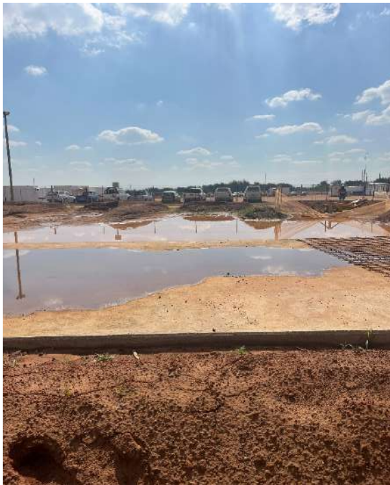
Figure 21: Vehicle Maintenance Slab
