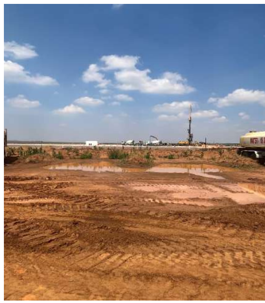
Figure 6: Water damming at parking area
