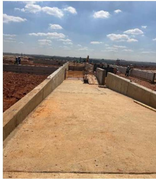
Figure 16: Silt Trap under Construction
