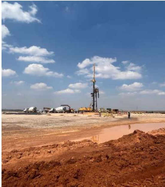
Figure 5: Water damming near shaft construction area
