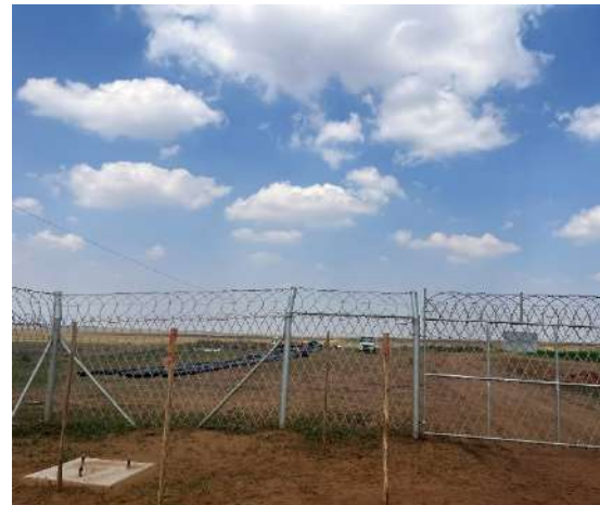
Figure 14: Construction of pipeline
