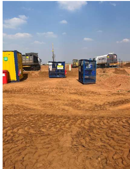
Figure 22: Chemical Storage at Jedd Civils' Laydown area
